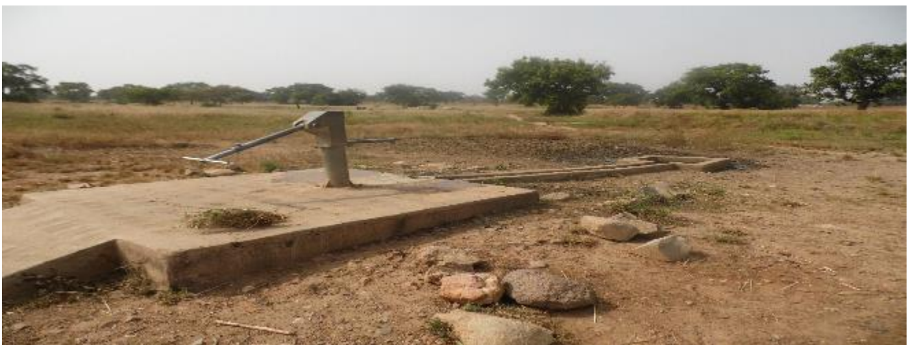
Plate 4-6: Borehole near Project Site
